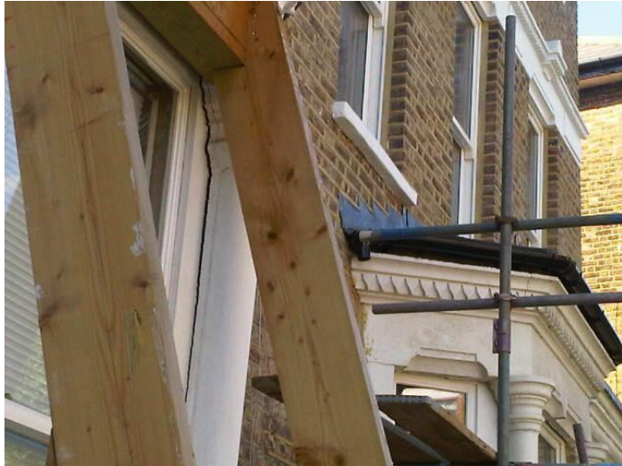
Emergency structural support in South Hill Park (left) and in Christchurch Hill (right) caused by basement developments
