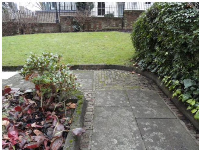
Some of the retained brickwork and materials
