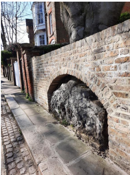
The wall of Grade II-listed 1 Cannon Place NW3
