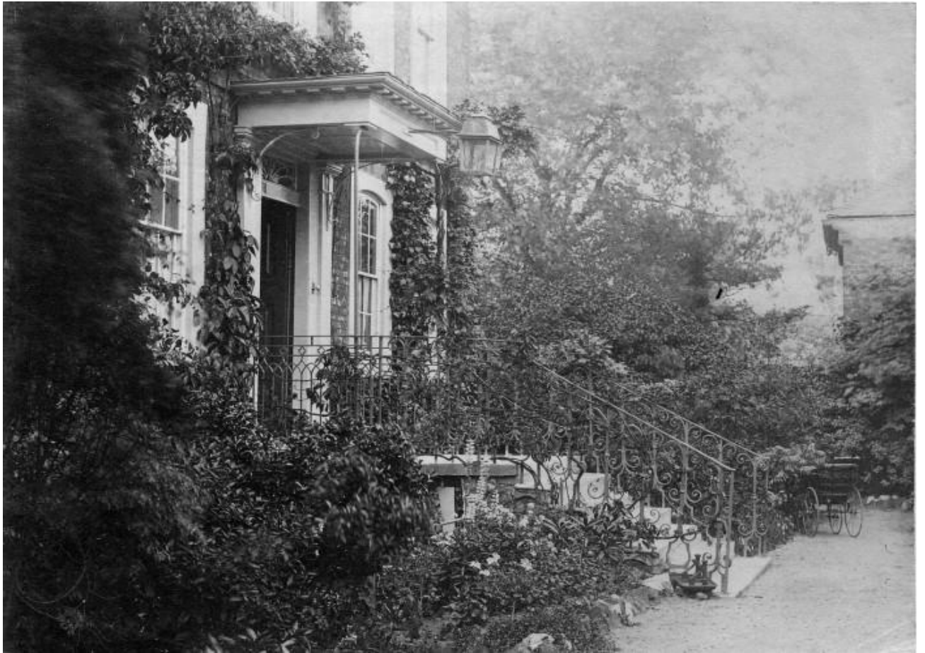
c1884-97 Burgh House front steps
